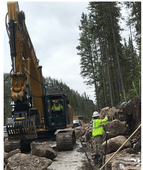
Road repairs in Yellowstone National Park. (Credit: The Pew Charitable Trusts)
